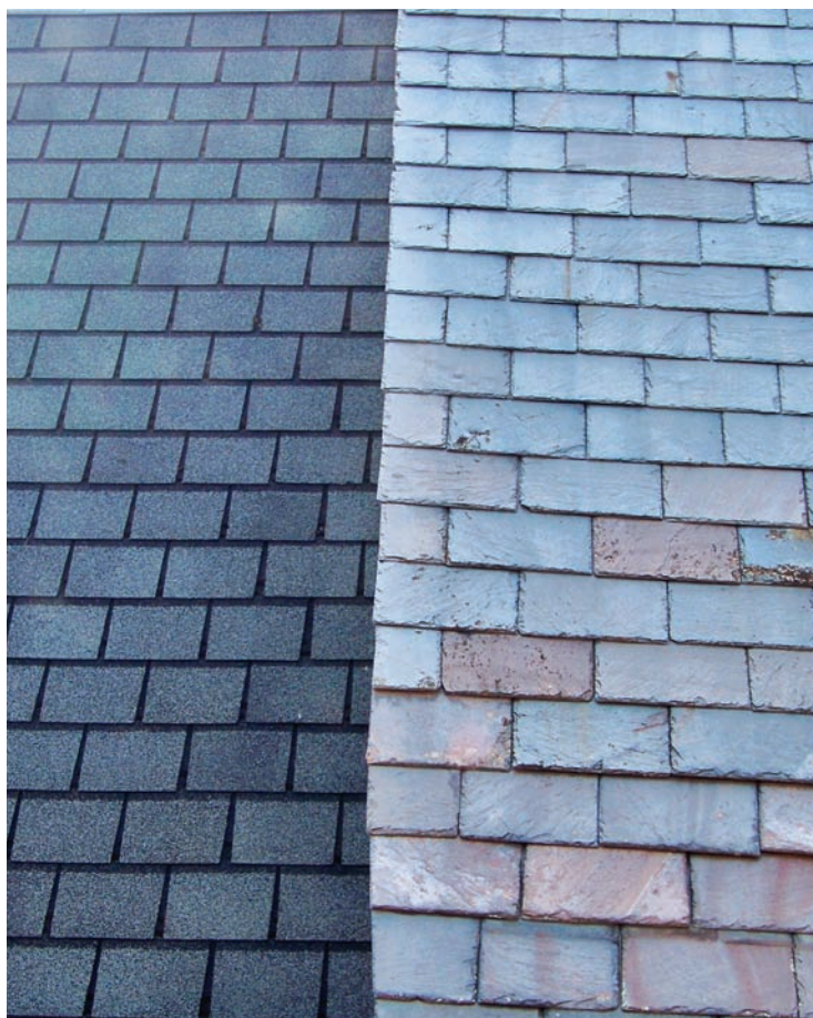
Above: Hatteras asphalt shingles by CertainTeed on Holy Trinity Episcopal Church in Swanton. Natural slate is at right. In photo at right, natural slate is at left.
