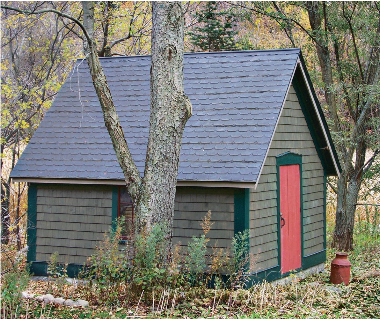
W.F. Norman produced a similar galvanized steel chamfered slate as on this 1800s cottage.
