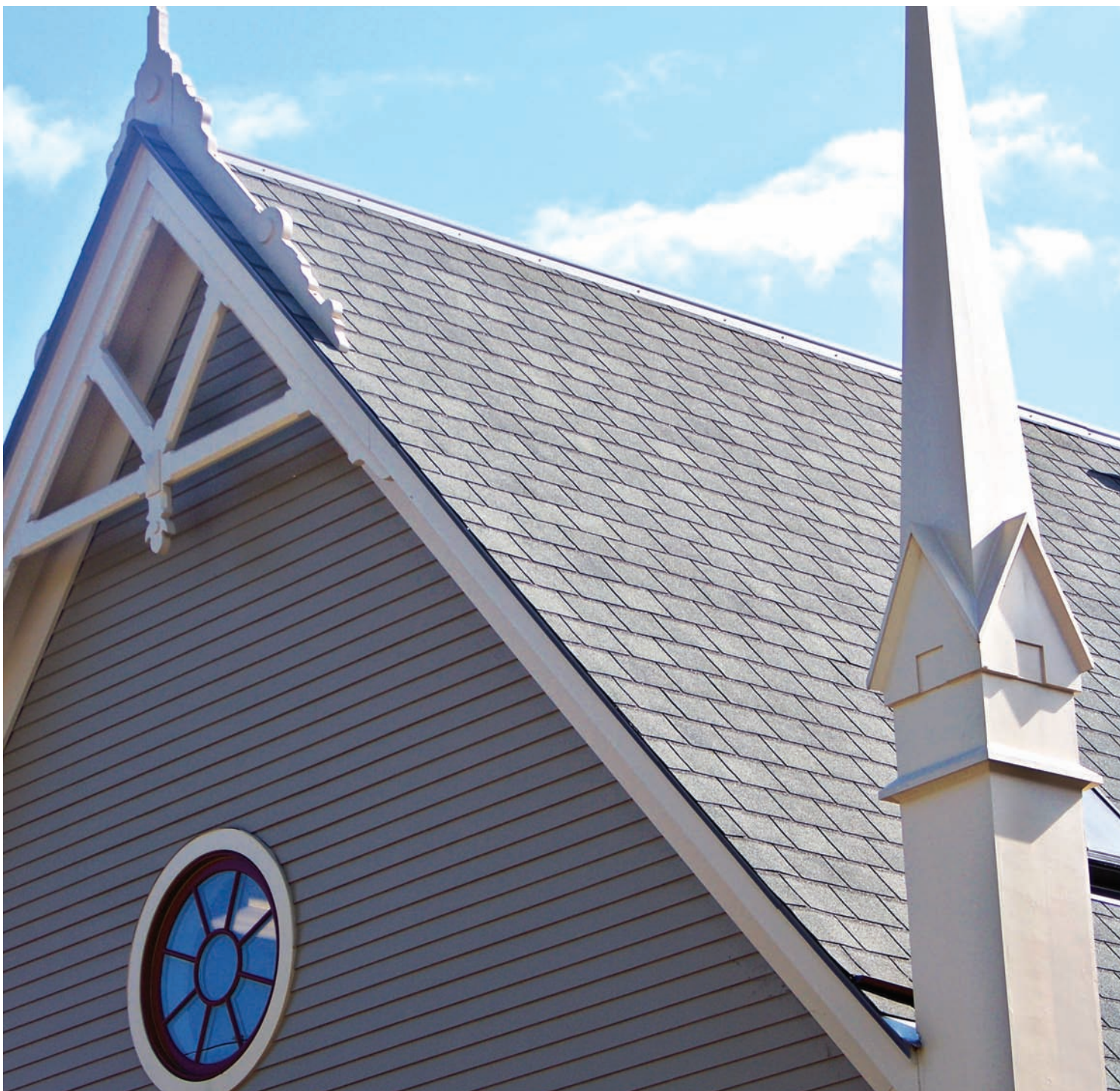
Hatteras asphalt shingle by CertainTeed on Holy Trinity Episcopal Church in Swanton.
