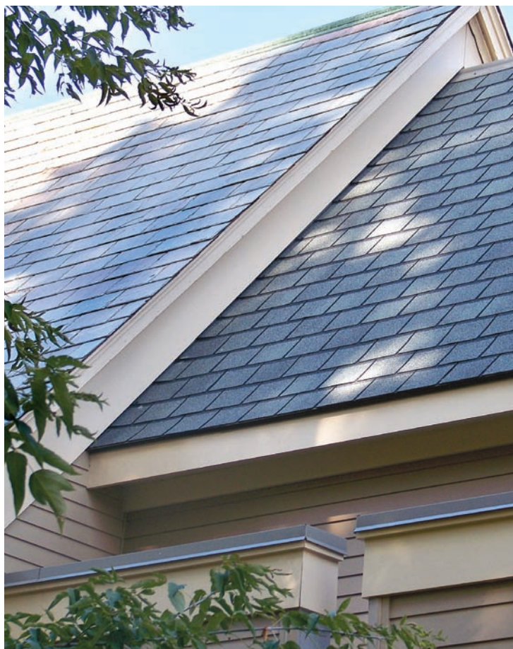
Above: Hatteras asphalt shingles by CertainTeed on Holy Trinity Episcopal Church in Swanton. Natural slate is at right. In photo at right, natural slate is at left.
